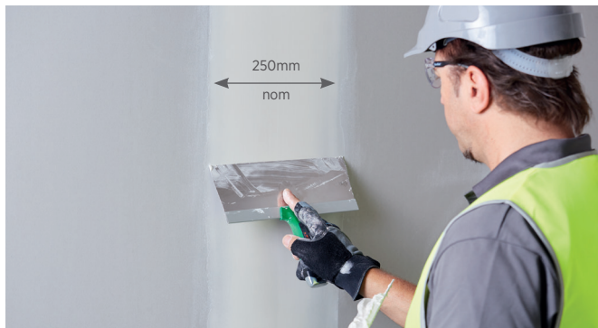
Step 5 Finishing coat
