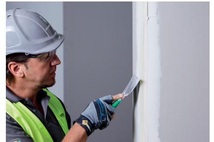
Step 1 - Alternative Flex metal tape
