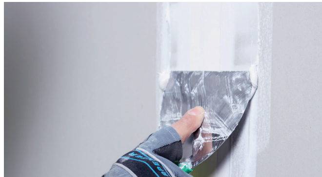
Step 4 First coat - Skim coat over tape
