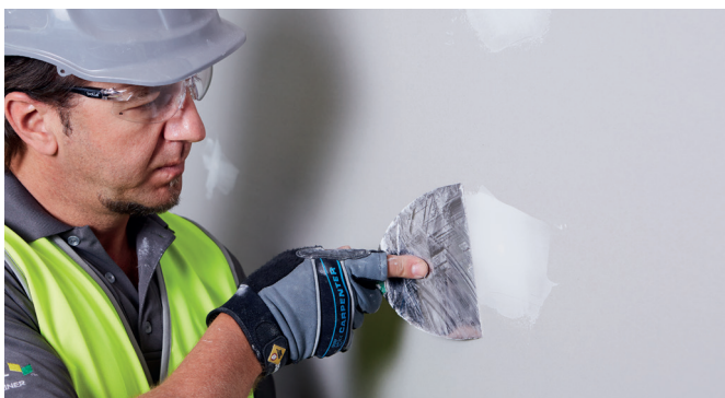
Applying 3 separate coats of joint compound over screw fixings
