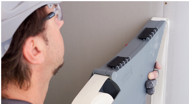
Step 3 First coat - Apply the tape and compounds along the joint
