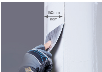
Step 2 Apply first coat to both corner faces
