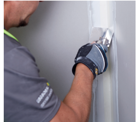
Step 3 First coat - Skim coat over tape
