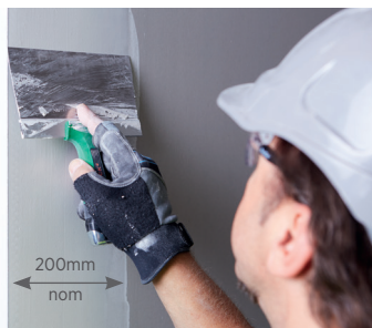
Step 3 Apply second coat to corner faces
