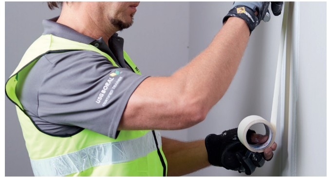
Step 2 First coat - Bed tape
