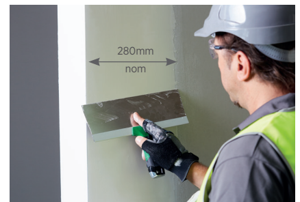
Step 4 Apply third coat to corner faces
