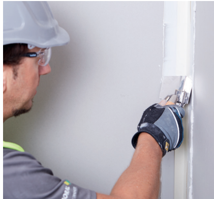
Step 2 First coat - Fold and bed tape
