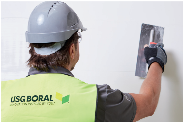
Application of joint compound over square edge joint
