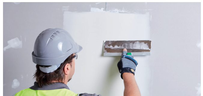
Step 1 Finishing coat for square edge joints
