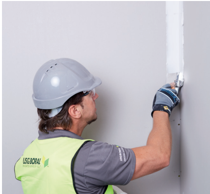
Step 1 First coat - Apply base compound
