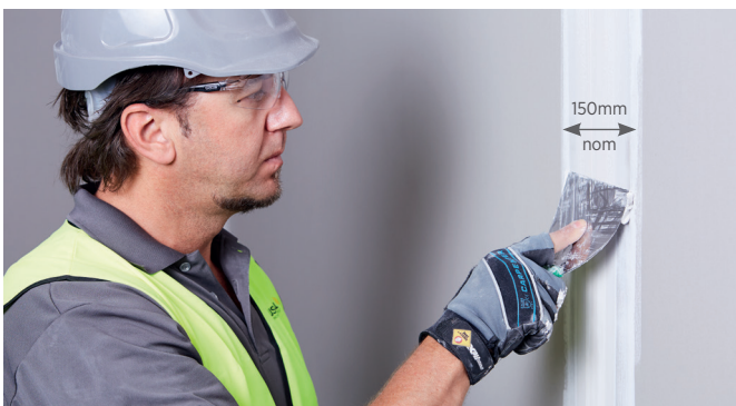
Step 3 First coat - Skim coat over tape
