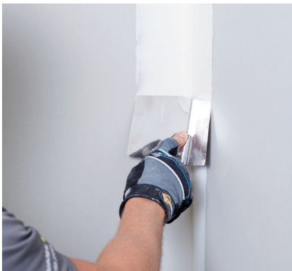
Step 4 Apply second coat
