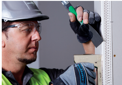
Step 1 - Alternative Plastic corner bead
