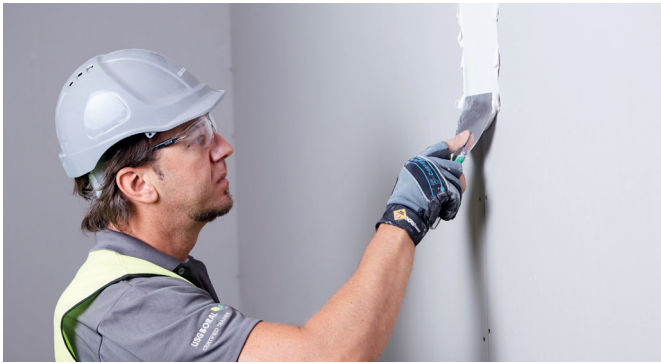
Step 1 First coat - Bedding compound
