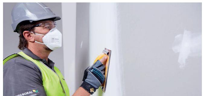
Step 3 Dry sanding of square edge joints
