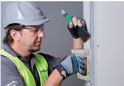
Step 1 - Perforated metal angle Cut angle and fix to sides of corner @ 300mm ctrs
