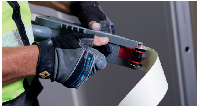
Step 2 Adjust the nozzle to ensure at least 1mm of compound is in under the tape
