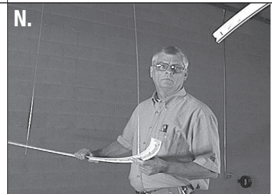
N. Install the next main tee segment. Refer to the ribbon drawing to select the correct segment.
