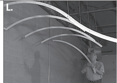
L. Continue to install the flush-cut main tees until all of the tees are installed at one end.
