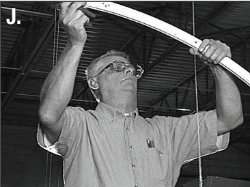
J. Install the flush-cut end of the main tee.
